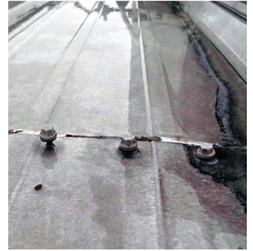
Loose or Missing Fasteners
